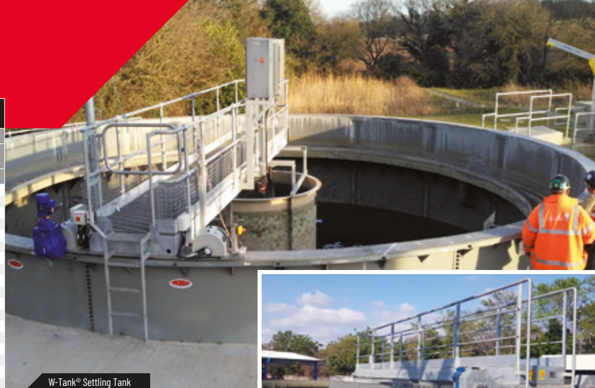
W-Tank® Settling Tank
